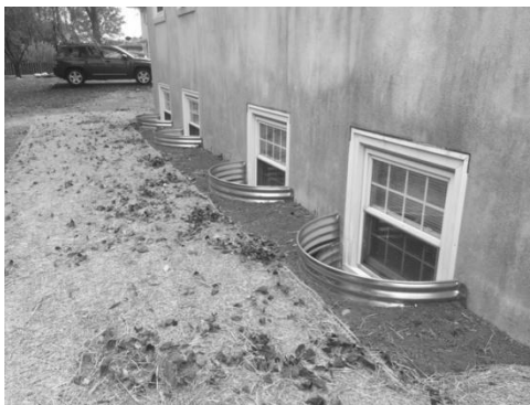
Regrading of landscape and raised window wells to eliminate water in basement
